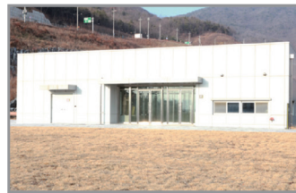
Chemical, biological and radiological (CBR) disaster experience center
